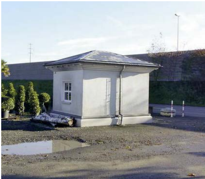
Pumpwerk Gütli in Widnau
